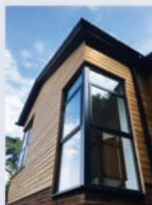
A recently completed project in Hurstpoint
